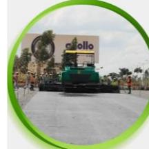
60 lane-kms of road is completed using waste plastic
